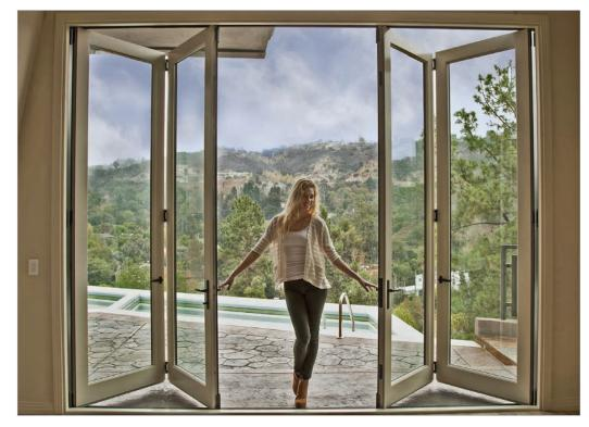
and hinged together to slide accordion-style and stack against one edge of the opening or the other.
