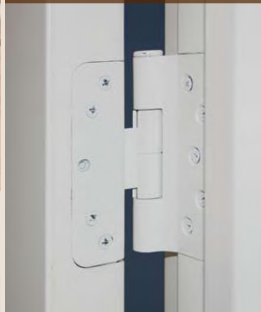
Four-way Adjustable Hinge
